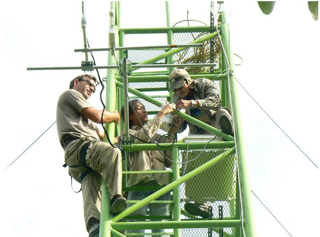
Installation of CO 2 /H 2 O analyzer (Licor-7500)
