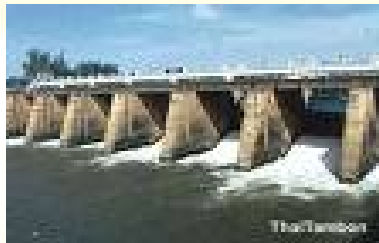
Mae Klong Dam 12.0 MW
