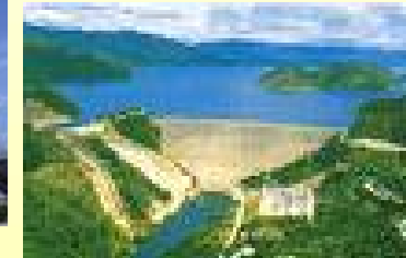
Kwae Noi Dam 30.0 MW
