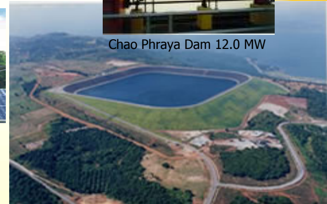
Lam Takong Pumped Storage 500 MW
