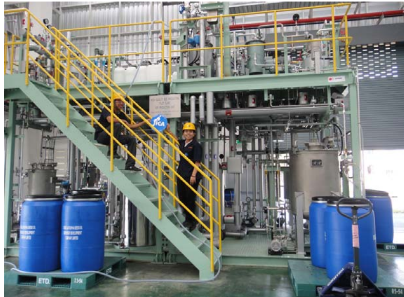
BDF Production Unit (1.0 ton-BDF/day)
