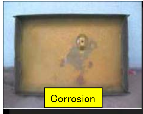
Fuel tank (source: Fuel Policy Subcommittee)
