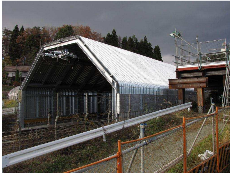
Tunnel Entrance Hood
