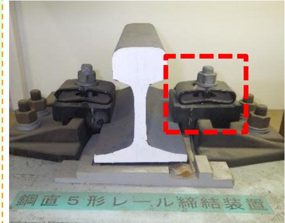
Steel bridges (Type 5 for bridge)
